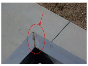
+ East corner welding is incomplete (tacked only) at the front exposed structural steel mounting bracket behind area shown in photo - Attention.
